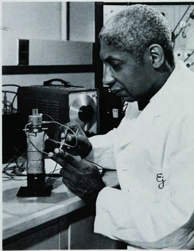
and audio acoustics and vibration. At left is a small (1.8 meter 3 ) anechoic chamber for measuring loudspeaker frequency response. At right Earle Jones calibrates an accelerometer for use with a transducer-shaker system.
