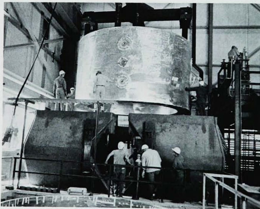
WORLD'S LARGEST SUPERCONDUCTING MAGNET is lowered into its steel frame at Argonne National Laboratory. The 110-ton magnet will produce an 18-kG field for the laboratory's 3.7-meter bubble chamber, whose usable volume is 20 m 3 . The Mirabelle chamber nearing completion at Serpukhov is longer (4.5 m), but its usable volume is only 6 m 3 .
