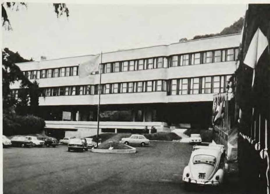
NEW HEADQUARTERS, provided by city of Trieste at $1 per year, looks down on Adriatic from a hillside in Miramare, about 6 km north of the middle of Trieste.
