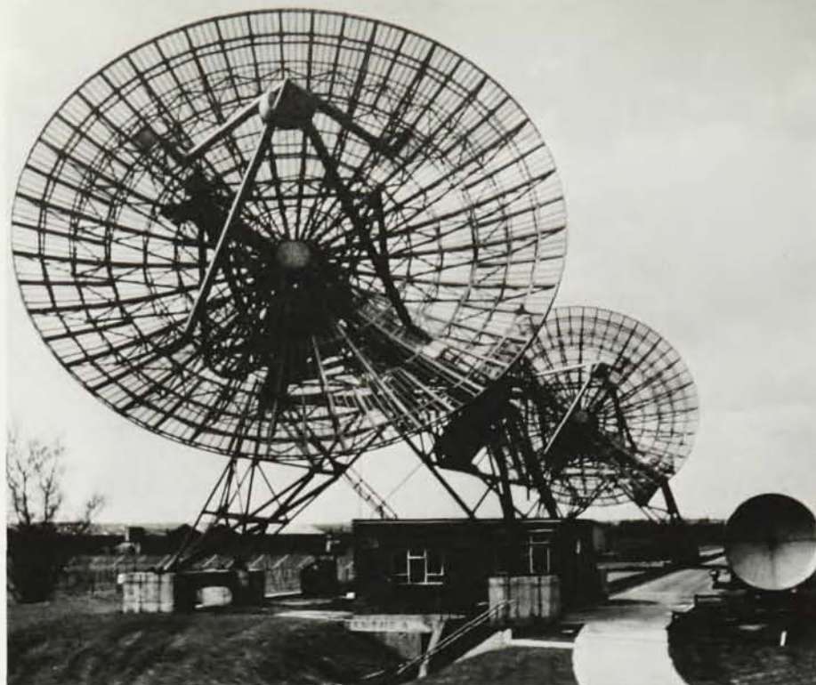
PORTION OF CAMBRIDGE 1-MILE INTERFEROMETER used to determine accurate location of CP 1919. Two of the three dishes are shown. The more distant of the two moves on railroad tracks. Solid dish is German World War 2 relic. —FIG. 1
