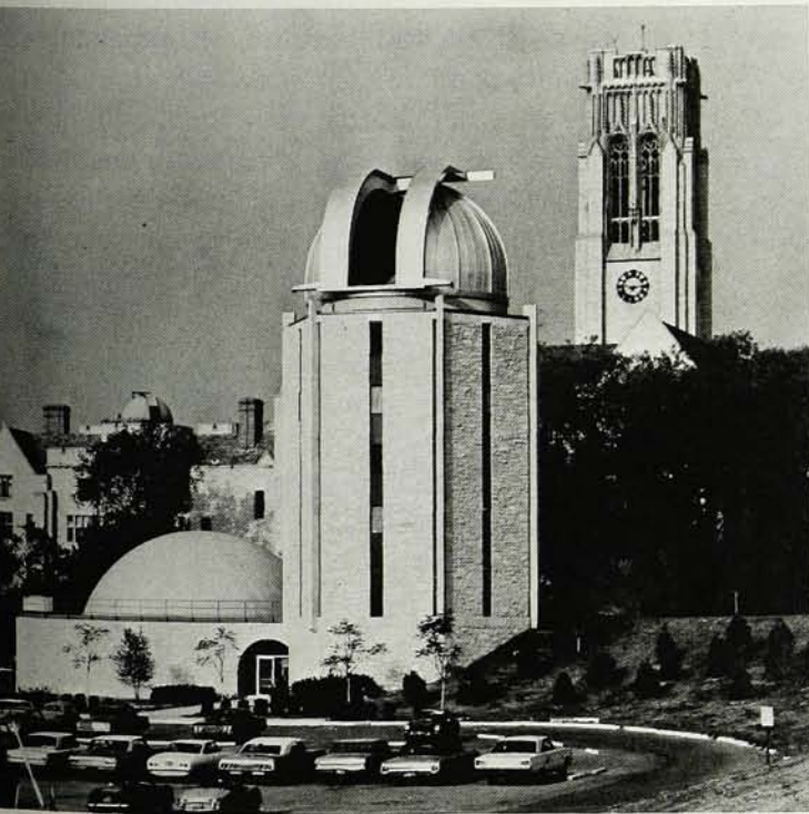
TOLEDO TELESCOPE has all CER-VIT optics; so images are limited only by diffraction and atmospheric distortion. Hollow pier will hold equipment for high-dispersion spectroscopy.
