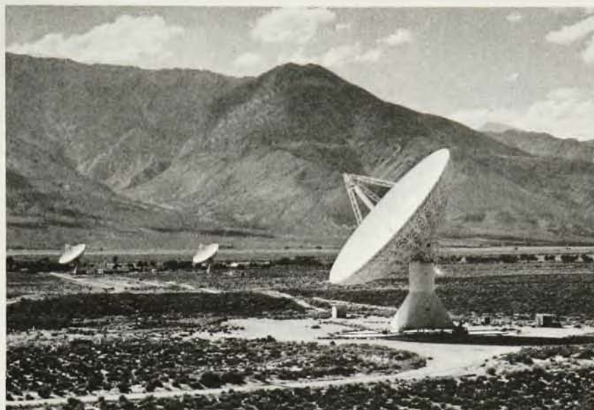
NEW 39.6-METER RADIO DISH at Owens Valley in California was dedicated 18 Oct. The $1.7-million instrument is the first in a proposed array of eight similar instruments to be mounted on rails in the shape of a cross with baselines of 4875 and 2750 meters. A special panel of the National Science Foundation has given the overall project high priority. In the background are two older 27-meter dishes that form a smaller interferometer on their own rail system 1065 meters from the proposed crossed array; these will be linked to the 39.6-meter antenna to form an interferometer with a much longer baseline. Present emphasis at Owens Valley is on interferometric studies of radio spectral lines, mapping the distribution of gas in our own and other galaxies.
