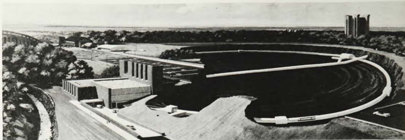
CUTAWAY VIEW OF THE CORNELL SYNCHROTRON shows the tunnel 13 meters below the athletic field. The straight tunnel across the diameter is for utilities and is also an escape route to the surface. Laboratory building is above ground level in scenic Cascadilla Gorge. —FIG. 1
