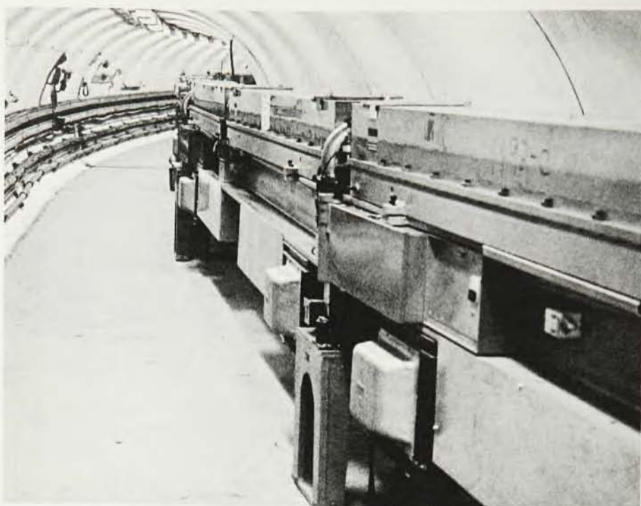
INTERIOR OF THE SYNCHROTRON TUNNEL. Magnets are inside the rectangular vacuum chamber on top of the support beams, and capacitors and biasing choke transformers are mounted under the beams. Tunnel diameter is 3 meters. —FIG. 4
