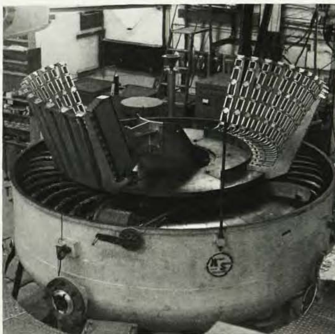
MIT MULTIPLE-GAP spectrograph set in large vacuum tank. —FIG. 6
