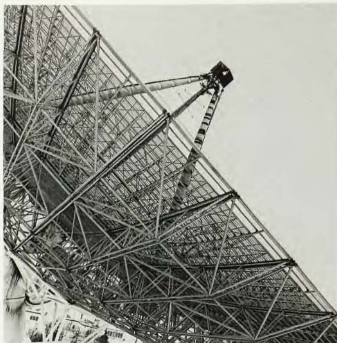
FEED MECHANISM of 84-ft dish for studies of ionospheric scintillations. —FIG. 3
