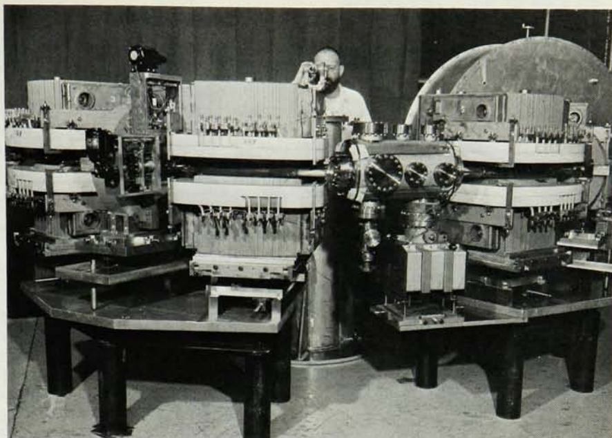
MURA ELECTRON-POSITRON STORAGE RING: Preliminary assembly.
