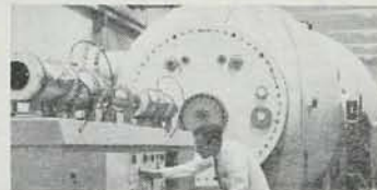
MP Tandem accelerator being installed at Atomic Energy of Canada Ltd. Chalk River Laboratories achieved 15 MV terminal voltage during initial test of the electrostatic structure.
