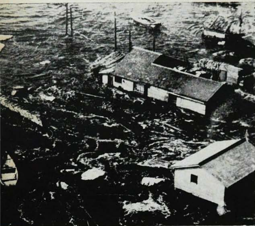
TSUNAMI RUNUP. On 4 March 1952 a wave caused by the Tokachi-oki earthquake reached a height of about 3.4 meters above normal tide at this village on Hokkaido.
