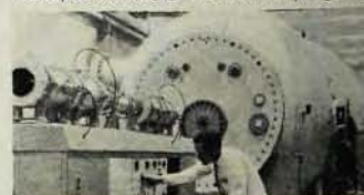
MP Tandem accelerator being installed at Atomic Energy of Canada Ltd. Chalk River Laboratories achieved 15 MV terminal voltage during initial test of the electrostatic structure.
