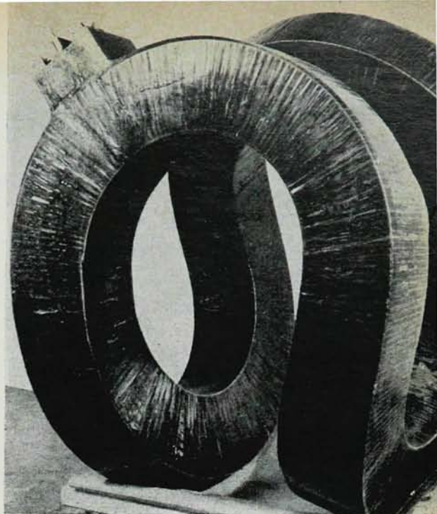
BASEBALL-SEAM COILS used at Livermore to produce minimum- B field for experiments on plasma containment and stability. Diameter is 1 meter.
