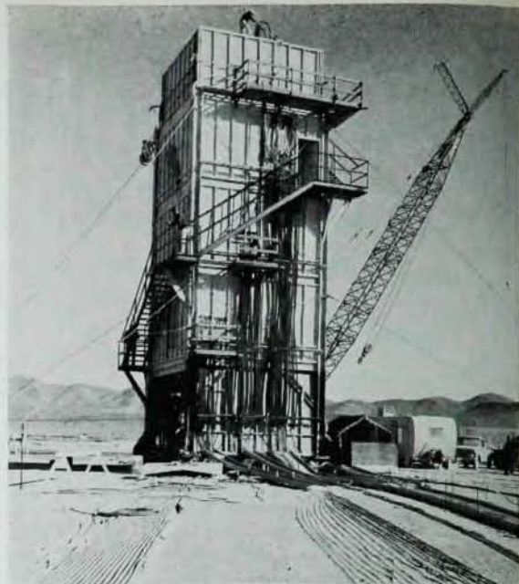
Fig. 2. Photograph of the instrument tower; its dimensions were 17 x 17 x 50 feet.
