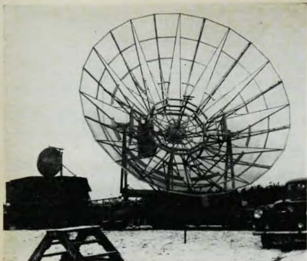
The transportable 25-ft dish in Yorkshire. With Mark I at Jodrell Bank, it forms an interferometer of maximum baseline 180 000 \lambda . (H. P. Palmer)
