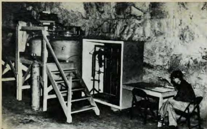
The Davis neutrino observatory in the Barbarton (Ohio) mine, 2300 ft underground. The two 500-gallon tanks are filled with perchloroethylene ( C_2Cl_4 ). Neutrino radiation transforms ^{37}Cl into radioactive ^{37}Ar .
