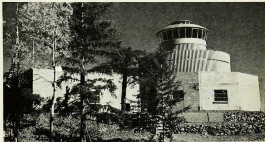
Laboratory building has two levels of observation deck and a rotating cupola on top which makes horizon scanning possible in all directions from fixed indoor instruments
