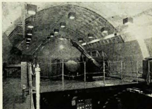
Fig. 4. View of PHERMEX showing electron-gun pulser and injector encapsulated in a plastic bag filled with \text{SF}_6
