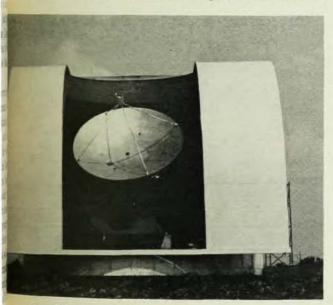
The 16-foot radio telescope at the University of Texas, designed to operate in the millimeter wavelength region, is housed in dome of type usually associated with optical telescopes.
