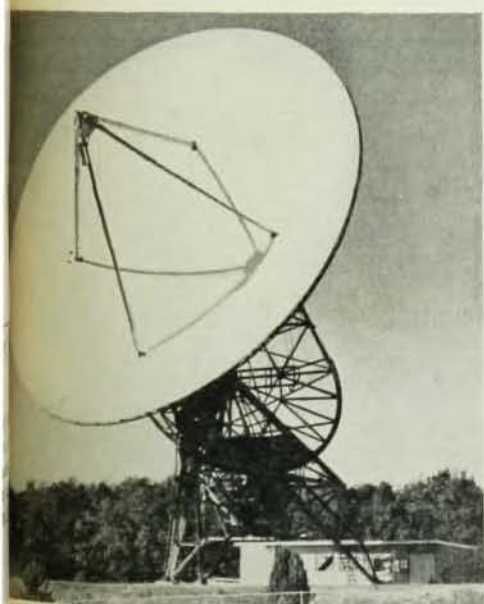
Fig. 3. Eighty-five-foot radio telescope at the University of Michigan is equipped with radiometers operating at 800, 8000, and 16 000 Mc/sec. This parabolic reflector has been used to measure the brightness temperatures of Mercury and Saturn and is now engaged in a survey of extragalactic radio sources. (University of Michigan Radio Astronomy Observatory Photo)
