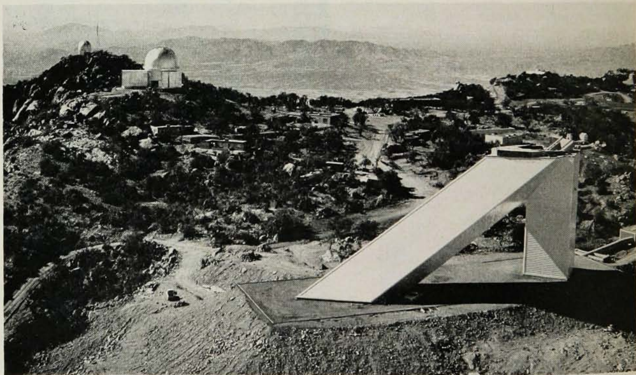
The above-ground structure of the new McMath Solar Telescope at Kitt Peak National Observatory. Domes for two of the Observatory's stellar telescopes appear in the background.
