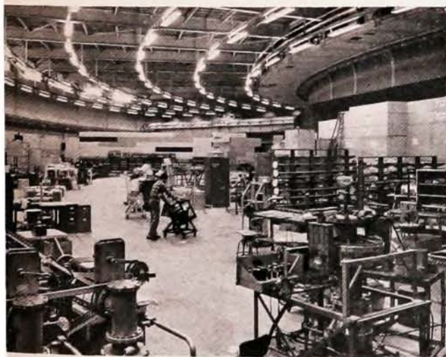
Experimental hall at Cambridge electron accelerator can accommodate as many as six simultaneous experiments, each involving a beam of high-energy electrons or photons.
