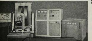
Illustrated: 12A-LI Electromagnet System. Includes magnet, "Line power supply, N.M.R. equipment and water-to-water heat ex anger. Pole face windings available to increase volume of uniformity
