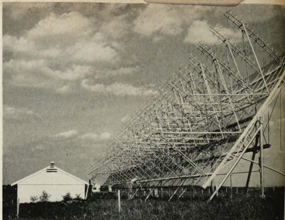
Fig. 1. Ohio State University 96-helix radio telescope antenna shown at right, has a beam approximately one degree wide in right ascension and eight degrees in declination at the frequency of 242 Mc.
