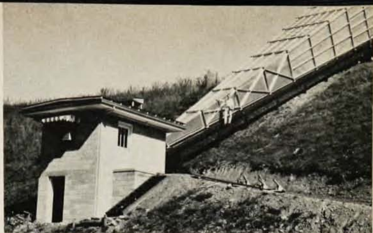
Above, Green Bank's 120-ft calibration horn antenna, used for accurate measurement of the intensity of radio radiation from Cassiopeia.
