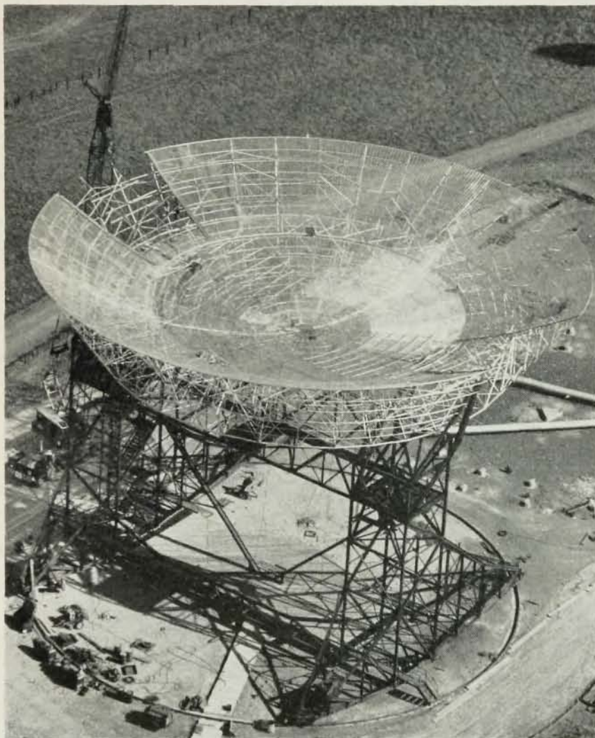
Aerial view of Stanford University's 150-foot radio telescope following installation.
