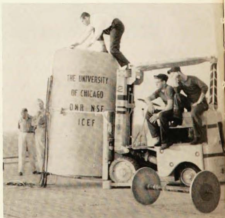
Balloon shroud lines are attached to top of emulsion gondola by David Haskin of the University of Chicago in preparation for launching. Project Director Schein can be seen standing at far left. (Photos courtesy NSF)
