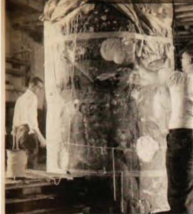
Battered gondola is patched up after first "Bravo" flight in preparation for second high-altitude exposure of 800-pound emulsion pack.
