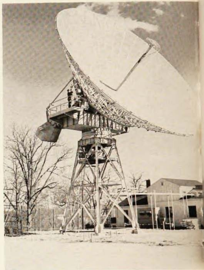
Diana, the 50-foot radar antenna at the Signal Corps Engineering Laboratories, Fort Monmouth, was constructed for use in tracking artificial earth satellites.
