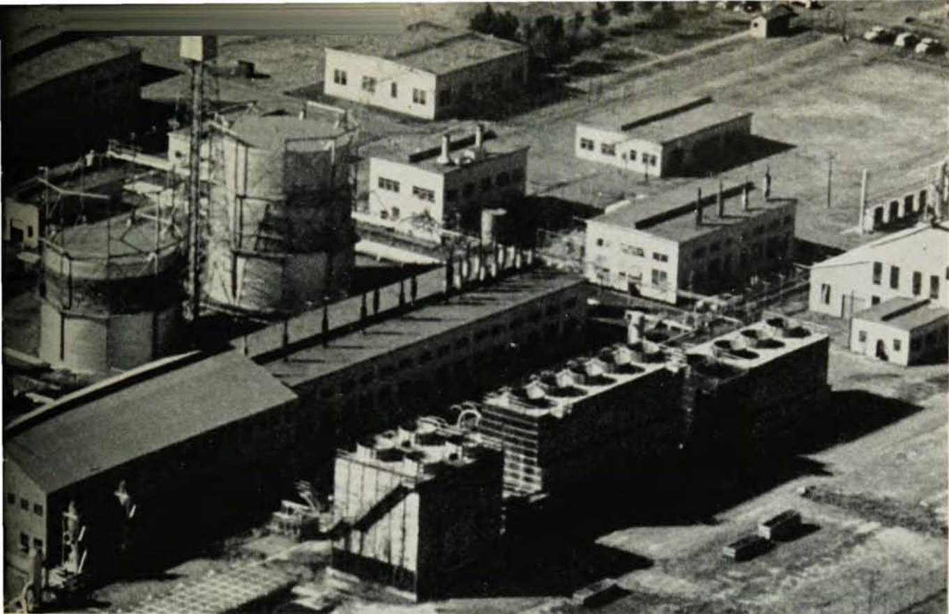
The largest plant for extracting helium is operated by the Bureau of Mines at Excell, Texas, about 30 miles north of Amarillo, and is about 7 years old. An addition completed in 1957 tripled its capacity. It processes natural gas containing about 0.9 percent helium gathered by a private gas producer for transmission to fuel markets.
