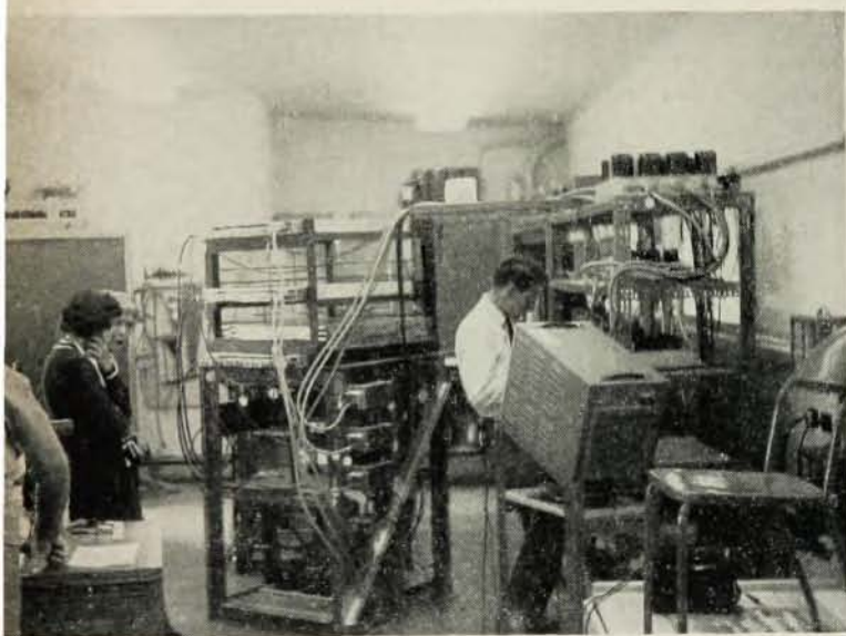
Interior of the Sulphur Mountain Laboratory, showing cosmic-ray meson telescope in center. Dr. Wilson is at the oscilloscope.
