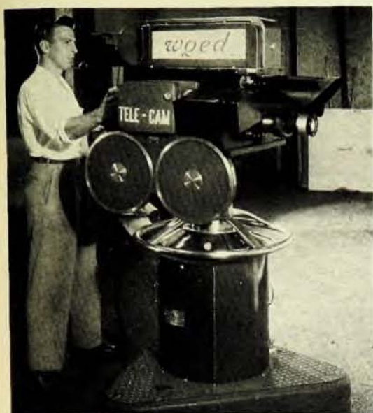
Fig. 2. Photograph of a cameraman with a Tele-Cam unit on a counter-weighted dolly.
