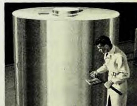
Nuclear Nutshell. Laboratory Reactor operates at 5 watts of power and produces more than 100 isotopes. It can be operated by one trained man.
