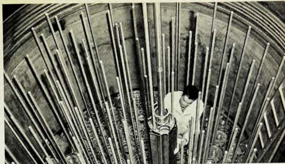
Reactor "heart". An AI technician installs zirconium "cans" containing the graphite moderator in the core of the Sodium Reactor Experiment. The use
