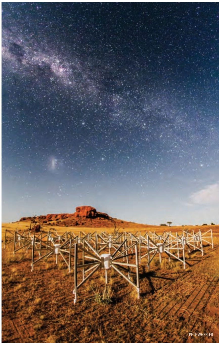
FIGURE 1. THESE ANTENNAS make up one of the 256 tiles in Australia's Murchison Widefield Array radio telescope, which was used in the discovery of ultralong-period radio transients—objects that pulse like cosmic lighthouses. Because of its location, the telescope is able to observe the southern celestial hemisphere.
