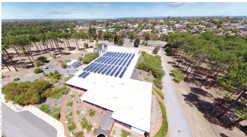
NEW SOLAR PANELS generate 118 kW at the Pawsey Supercomputing Research Centre in Perth, Australia. That is sufficient to power with net zero emissions a cooling system based on groundwater.
