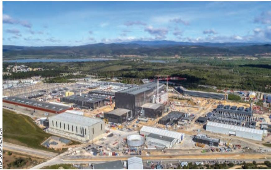
**AERIAL VIEW** of the ITER site in May 2021. The cryoplant, magnet power conversion facility, and electrical switchyard are located to the left of the tokamak complex and assembly hall at center. The heat-rejection plant and central offices are to the right.
