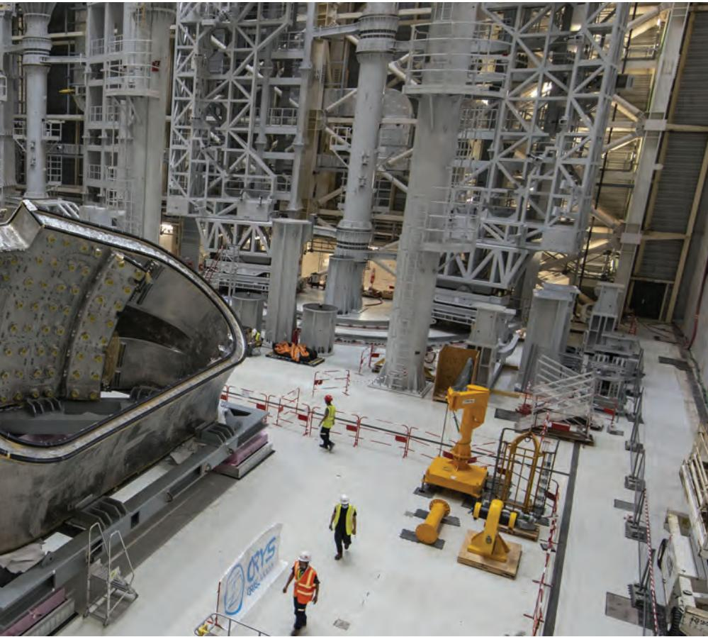
**A SECTION** of the ITER vacuum vessel, shown here at the ITER site in France, after its shipment from South Korea. When all nine sections are assembled, they will form the toroidal chamber that will contain the fusion plasma. The French nuclear regulatory agency halted assembly of the first two sections in January, after finding that misalignments caused by damage during shipment would prevent them from being properly welded.
