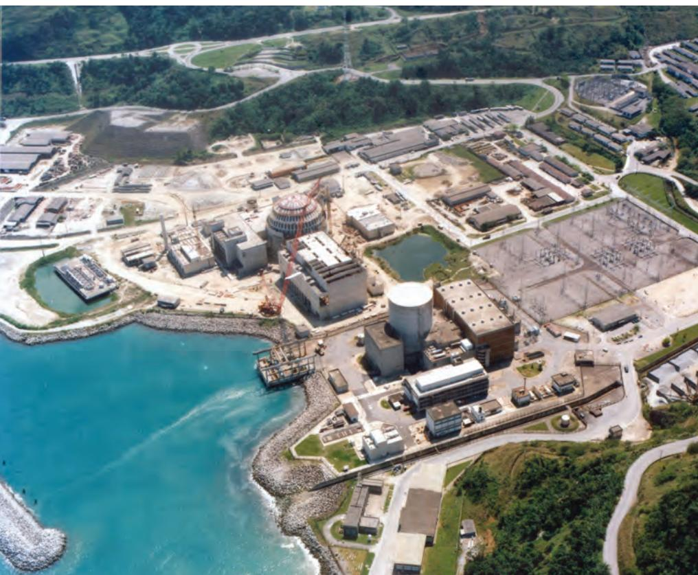
**FIGURE 4. THE ANGRA** nuclear power station, located in the southern part of the state of Rio de Janeiro. The only commercial facility in Brazil, it consists of two pressurized water reactors; a third is under construction. (Courtesy of FURNAS Centrais Elétricas/IAEA Imagebank/CC BY-SA 2.0.)
