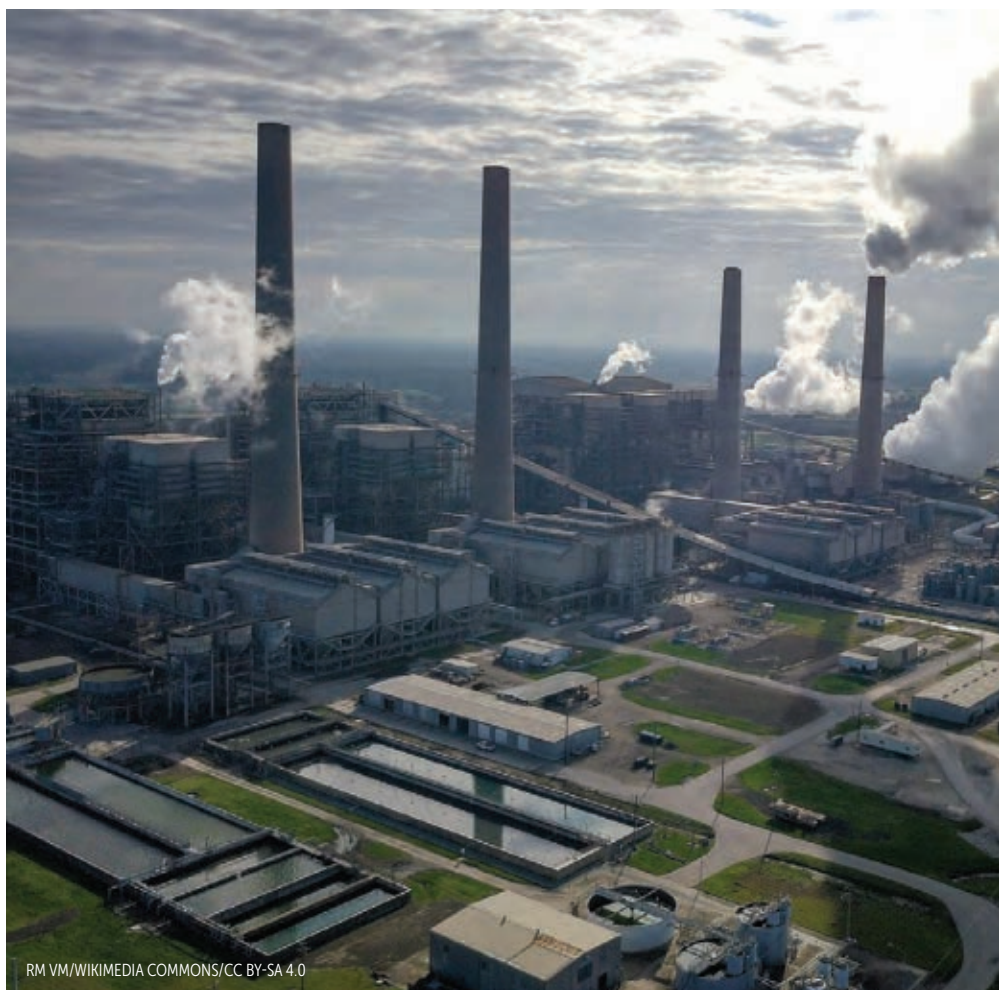
THE PETRA NOVA plant in Thompsons, Texas, was the only US power plant to successfully capture carbon dioxide from postcombustion at a commercial scale. The CO 2 was compressed and piped to an oil field for enhanced oil recovery. The system operated from 2017 until 2020, when low oil prices made capture uneconomic.
