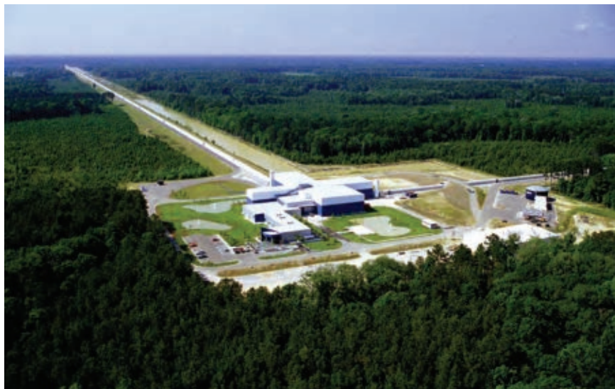
FIGURE 1. AT LIGO'S TWIN DETECTORS —this one in Livingston, Louisiana, and the other in Hanford, Washington—powerful laser light circulates in perpendicular 4-km-long arms. Through interferometry of the light from the two arms, researchers can detect changes in the arm lengths of less than 10^{-18} m. (Photo courtesy of Caltech/MIT/LIGO Lab.)
