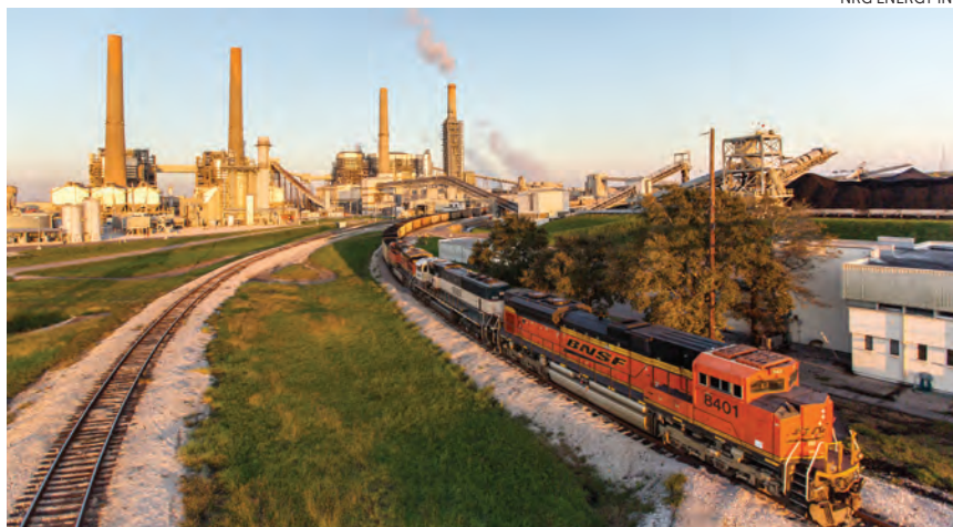
THE PETRA NOVA facility in Texas is the sole commercial fossil-fuel power plant in the US capable of capturing its carbon dioxide emissions. The retrofitted capture equipment was switched off in 2020 because of economic conditions, including a drop in demand for CO 2 used for enhanced oil recovery.
