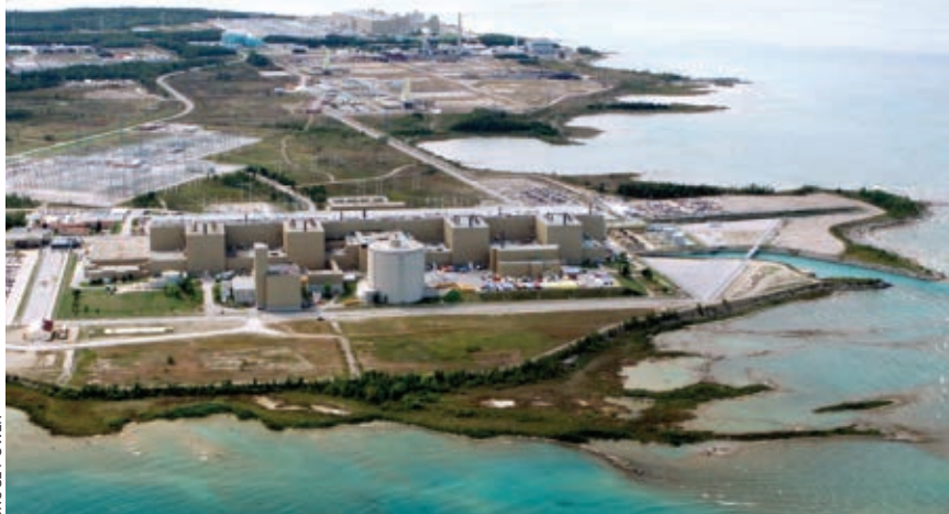
THE BRUCE NUCLEAR GENERATING STATION on Lake Huron is the largest nuclear power plant in North America. Its eight CANDU reactors produce 30% of Ontario's electricity. Four of the reactors are in the foreground; the others are visible in the background.
