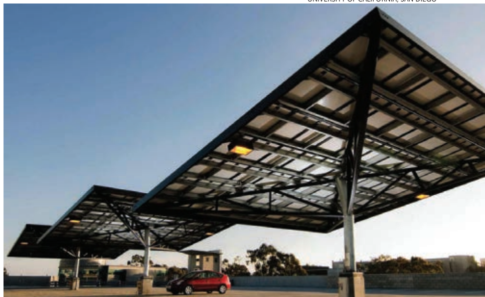
ONE OF 15 SOLAR POWER GENERATORS that will be part of a set of 2000 devices linked to form a power-use test bed at the University of California, San Diego. The test bed will allow the exploration of algorithms to better manage power grids.
