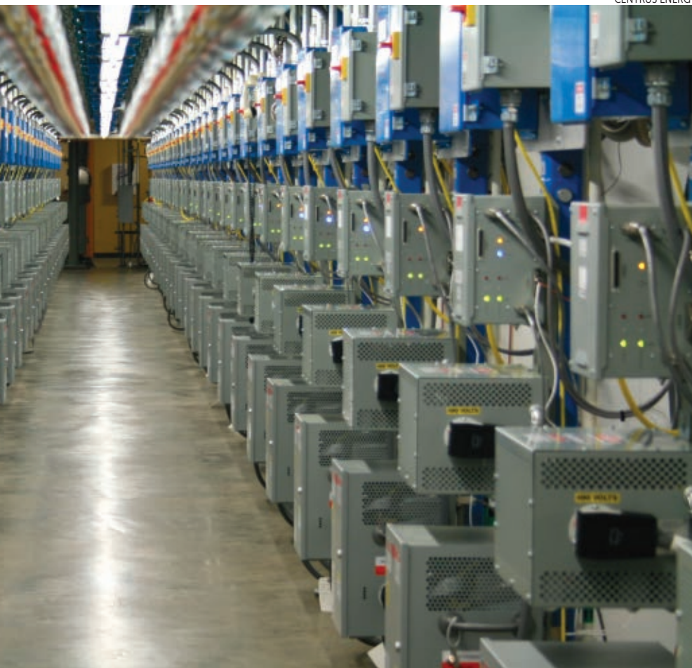
CENTRUS ENERGY'S 120-centrifuge uranium enrichment demonstration plant was in operation from 2013 to 2016 in Piketon, Ohio. The 12-meter-tall AC100M centrifuges have been decommissioned, but Centrus has continued developing the technology under contract with the Department of Energy.
