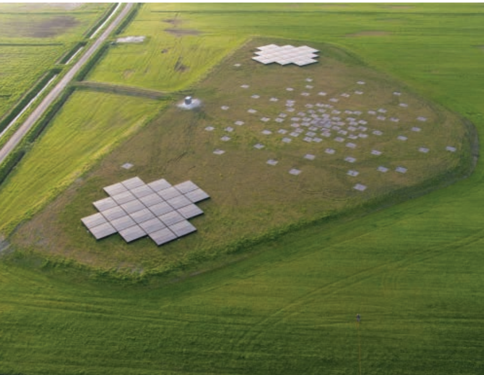
FIGURE 2. THE LOW FREQUENCY ARRAY (LOFAR) TELESCOPE is a collection of 25 000 individual dipole antennas distributed among 51 stations across Europe. One of the densely spaced Dutch stations is shown here. Each antenna in the center group—a metal pole with wire mesh underneath—detects low-band frequencies in the range of 10–80 MHz. The other antenna groups are housed in aluminum tile boxes and detect high-band frequencies in the range of 120–240 MHz. (Photo by © Top-Foto, Assen.)
