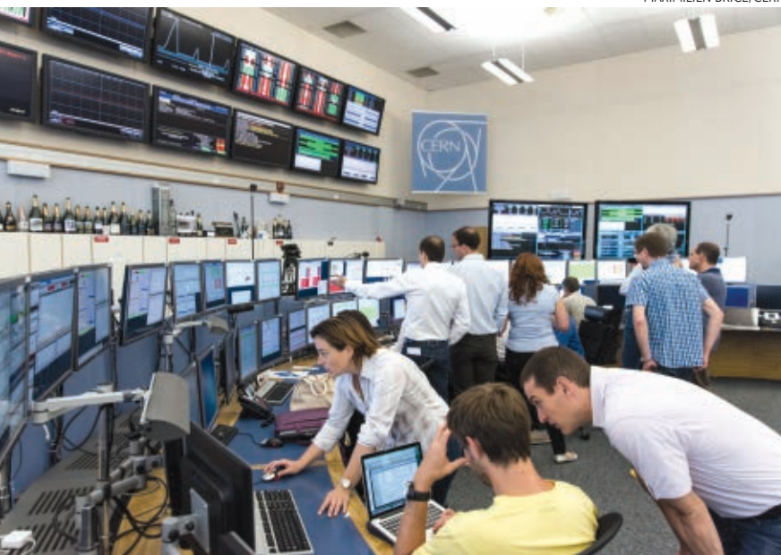
FIGURE 1. THE CERN CONTROL CENTER is made up of four “islands” in one big room. Each island has a circular arrangement of consoles and displays. They control the Large Hadron Collider (above), the Proton Synchrotron and Super Proton Synchrotron in the collider injection chain, and the technical infrastructure of the CERN accelerator complex.
